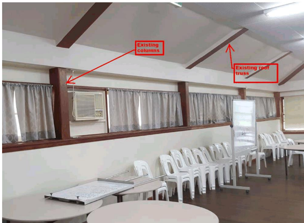
Figure 6.0 Location of columns inside club house completed in 1960 note the exposed column and truss bottom plate of roof truss.
